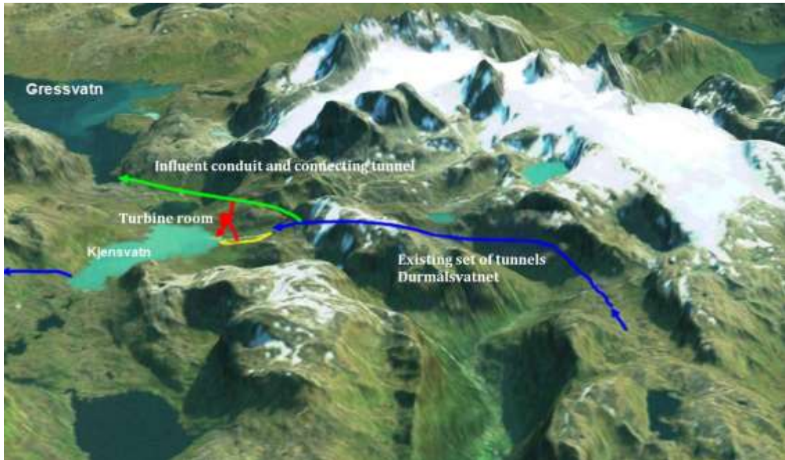
Pic. 1.: Picture of the newly constructed hydropower plant
